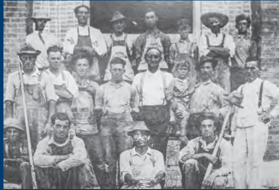
WM. Friede Construction Crew, circa 1898
