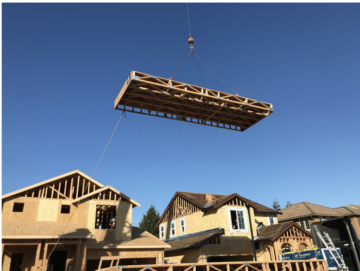
An Entekra floor assembly is hoisted into place. Entekra
