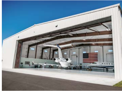
Nelson Family Holdings Hangar | Baraboo Silver Award: Pre-Engineered Building $1 Million to $2.5 Million
