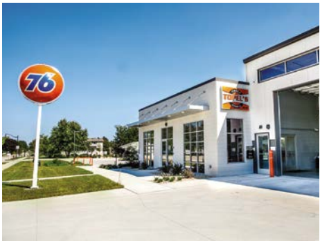
Topel's Service Center | Lake Mills Silver Award: Pre-Engineered Building Over $2.5 Million | Built on Merit Award
