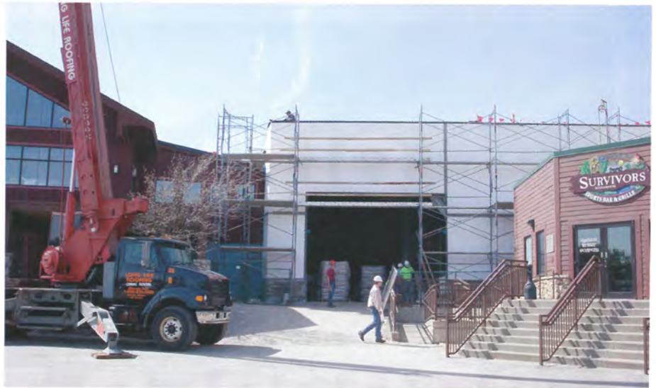
The only entrance into the work area is through the building being constructed that connects three previously constructed buildings. The Survivors restaurant entrance is also the main entrance for the water park and it also receives resort deliveries. Crews had to stage materials to allow parking lot access and coordinate equipment and material movement around guests and each other.
