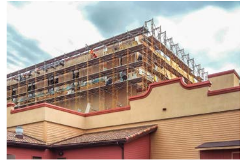
Left: A fabric cover over the interior scaffolding helped reduce the heat loss from within the waterpark. Exterior scaffolding was essential to replace the parapets and roof structure.
