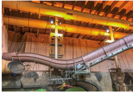
Left: A fabric cover over the interior scaffolding helped reduce the heat loss from within the waterpark. Exterior scaffolding was essential to replace the parapets and roof structure.
