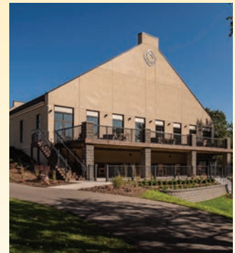
Glen Erin Golf Club Banquet Hall Gilbank Construction, Inc.
