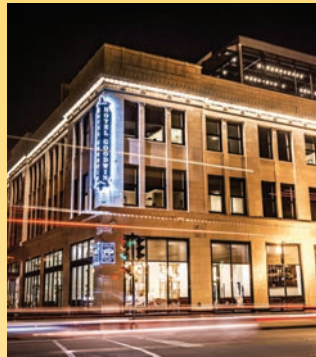
Hotel Goodwin | Velvet Buffalo Cafe / Corporate Contractors Inc.
