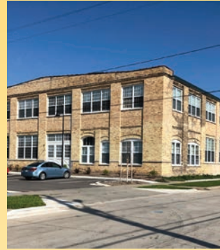
Waite Rug Place McGann Construction
