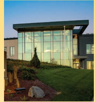
Illumina - New Research Facility Faith Technologies, Inc.
