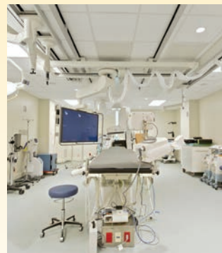
Saint Michael's Hospital - Nuc Med/Cath Lab / Ellis Construction
