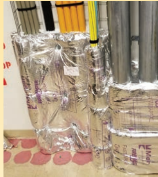
Children's Hospital T-ratings / Alpha Insulation and Waterproofing, Inc.
