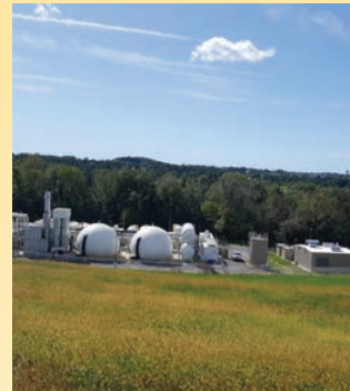
Dane County BioGas Facility Joe Daniels Construction Co., Inc
