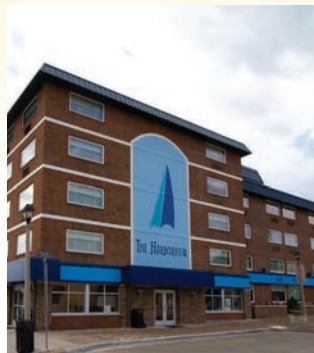
Harborview Hotel Remodel Northcentral Construction
