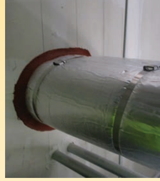
Froedtert Hospital Vertical Expansion / Alpha Insulation and Waterproofing, Inc.
