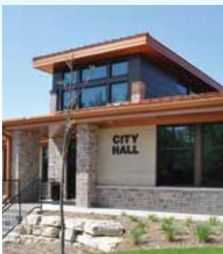
City of Baraboo Public Safety & Administration Building / Kraemer Brothers
