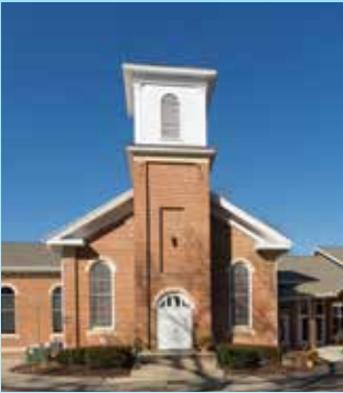
Fulton Church NCI-Roberts Construction
