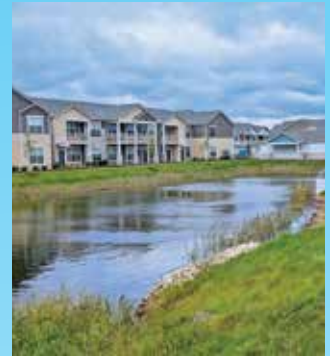
Springs at Sun Prairie Wondra Construction Inc.
