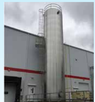
Masters Gallery New Plant HVAC & Refrigeration / Rohde Brothers, Inc.
