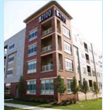
The 2100 Urban Residences Altius Building Company
