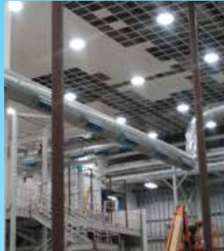
Duraform Lane Facility North American Mechanical, Inc.
