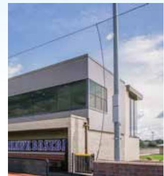
UW-Whitewater Athletic Complex Buildings / Gilbank Construction, Inc.
