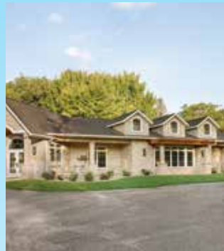
Welcome Center / Altmann Construction Co. Inc.
