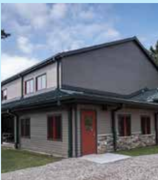
Camp Gray The Ark - Gymnasium Holtz Builders, Inc
