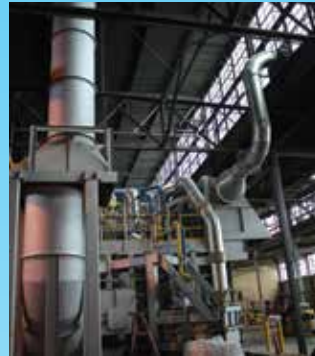
Skana Aluminum Co. Cast House Expansion / A.C.E. Building Service
