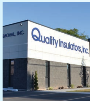
Quality Insulators, Inc., Keller, Inc.
