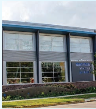
Reconstruction of the Madison Water Utility Operations Center, Joe Daniels Construction Co., Inc
