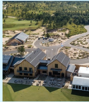
Sand Valley Golf Resort, Corporate Contractors, Inc.
