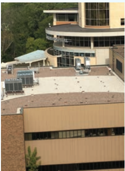
University Hospital Roof Replacement - H17-101, Pioneer Roofing, LLC
