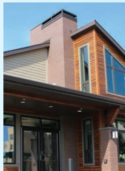
Shady Lane Assisted Living Expansion, A.C.E. Building Service
