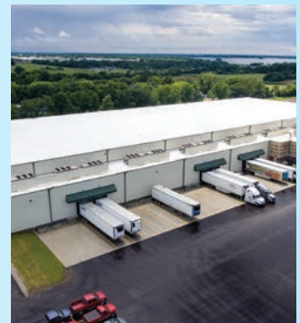
Beaver Dam Cold Storage, WDS Construction, Inc.
