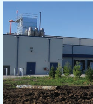
Greenfield Refrigerated Warehouse Facility, ESI Constructors, Inc.
